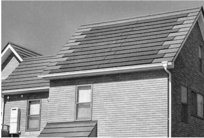
Figure 22.32 Prefabricated Japanese tilelike roof panel method with CdTe cells in Nie-ken (JA). Capacity of the system is 1.3 kWp. Reproduced with permission by MSK Corporation
