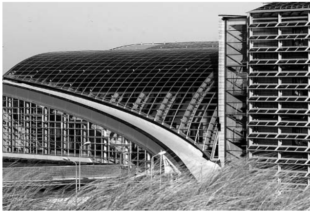
Figure 22.43 This building, at ECN in Petten (NL) has a 43 kWp PV system integrated into the conservatory roof. The conservatory acts as a parasol in front of the offices, thus eliminating the need for air-conditioning in a moderate climate. The building on the right side has a PV shading system (see caption on Figure 22.11). Reproduced with permission by BEAR Architecten T. Reijenga
