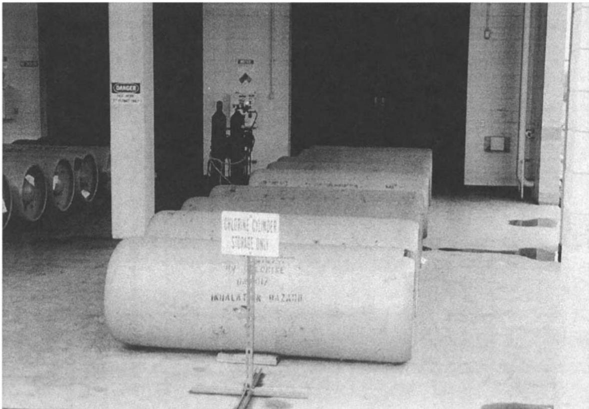
Photo 8.1 One ton chlorine tanks.
