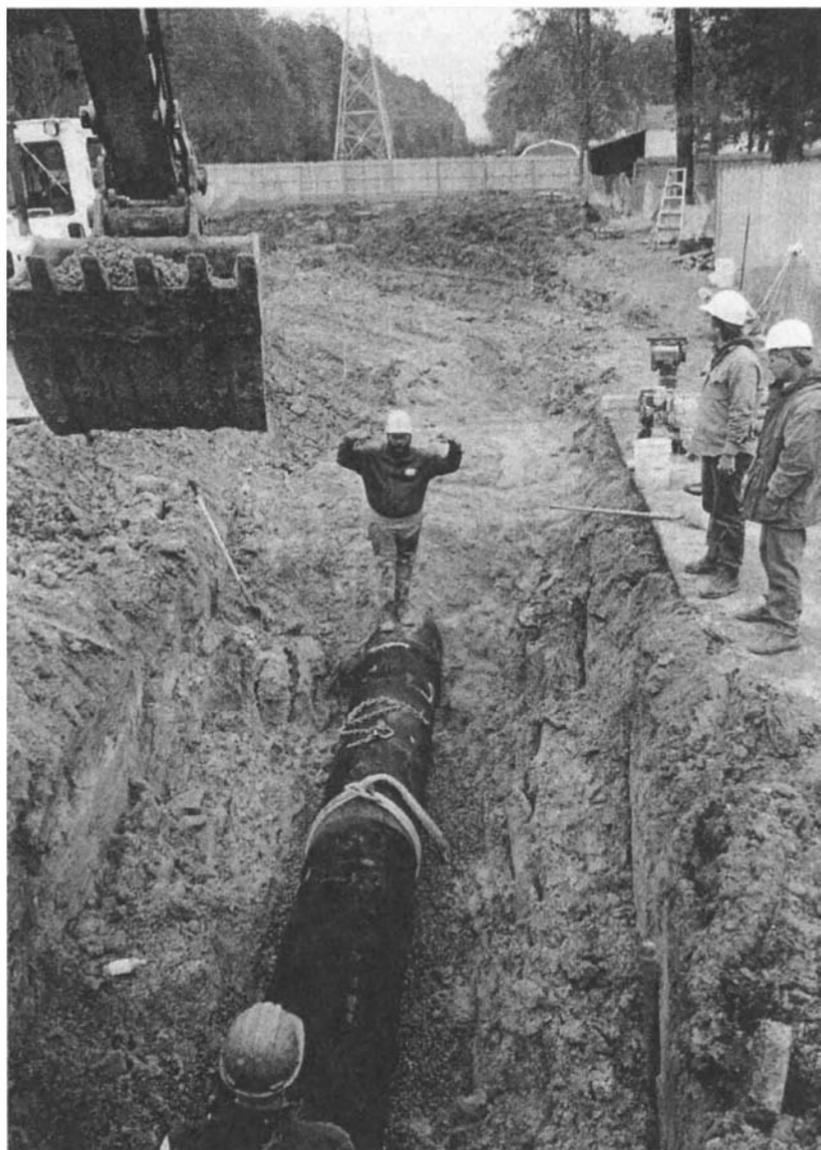
**Photo 13.4b** Replacing interceptor pipe.
