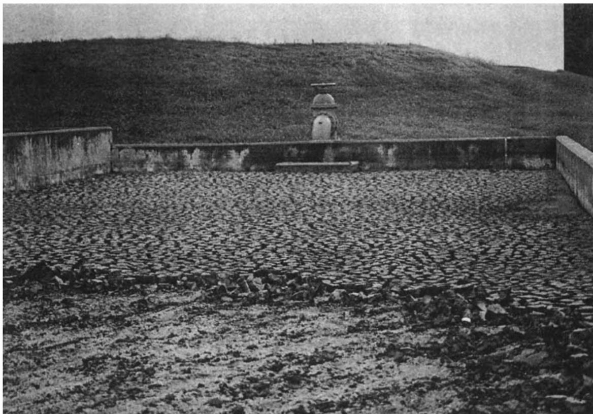
**Photo 24.4d** Sludge drying bed (process finished).
