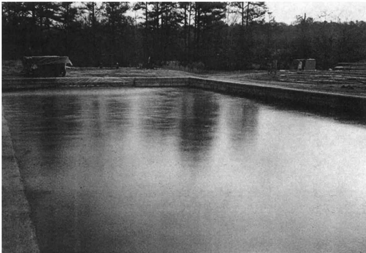
**Photo 24.4a** Sludge drying bed.
