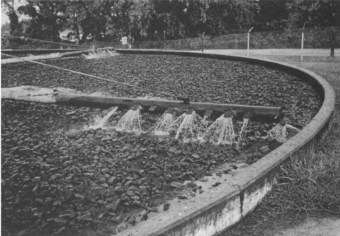
Photo 16.3 Trickling filter.
