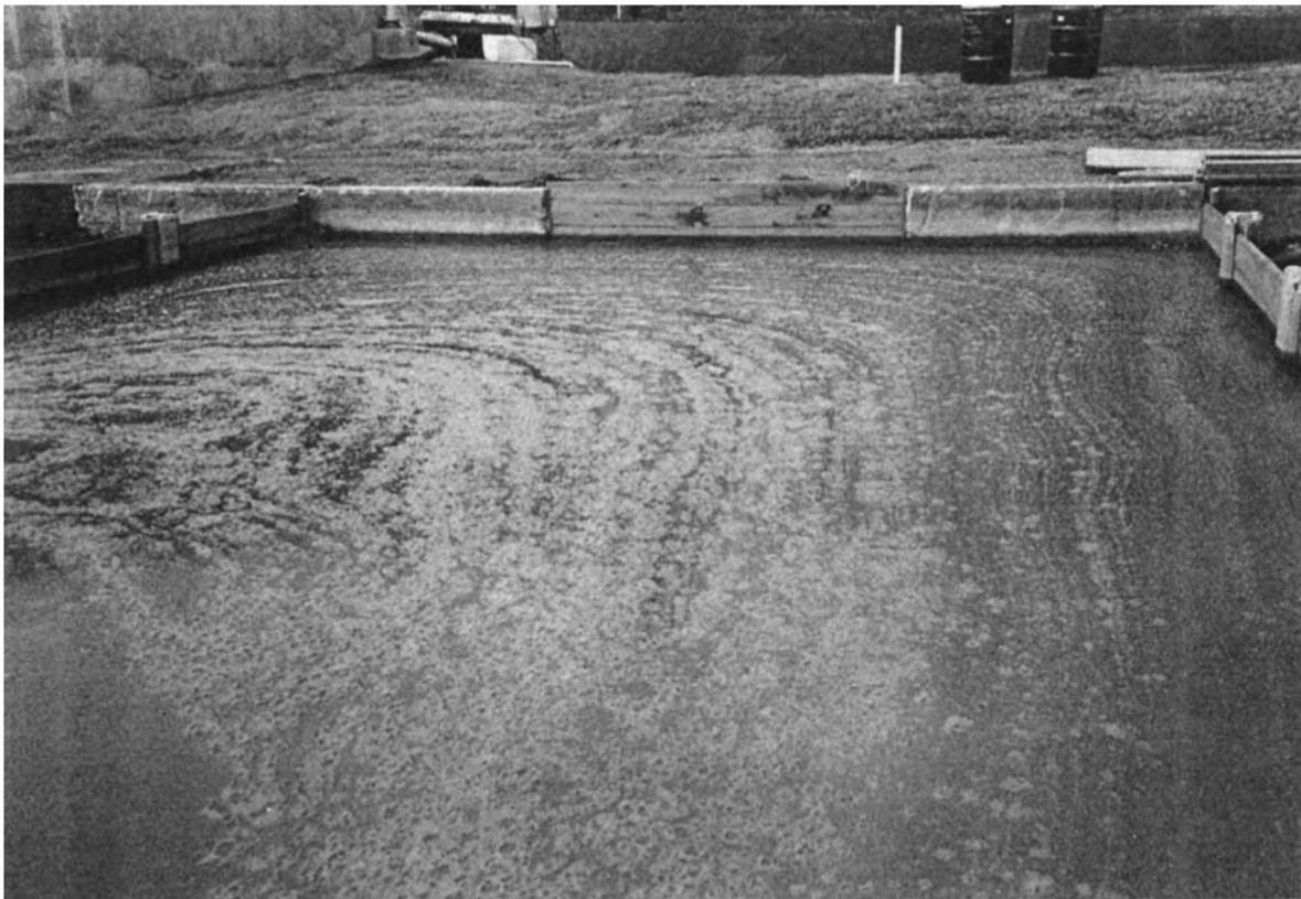
**Photo 24.4b** Sludge drying bed (drying in progress).
