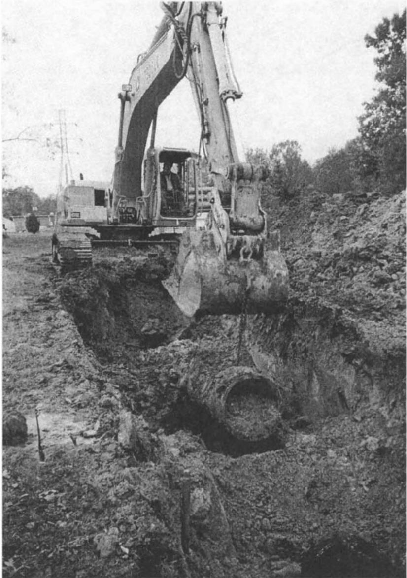
**Photo 13.4a** Removing broken interceptor pipe.
