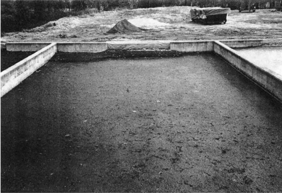
Photo 24.4c Sludge drying bed (drying in progress).
