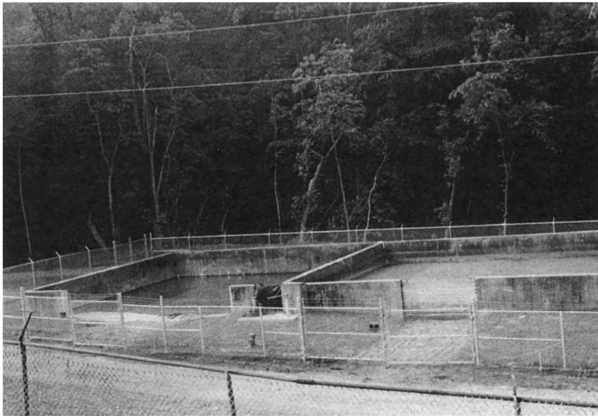
**Photo 22.1** Alum sludge drying beds, left side empty, right side full.
