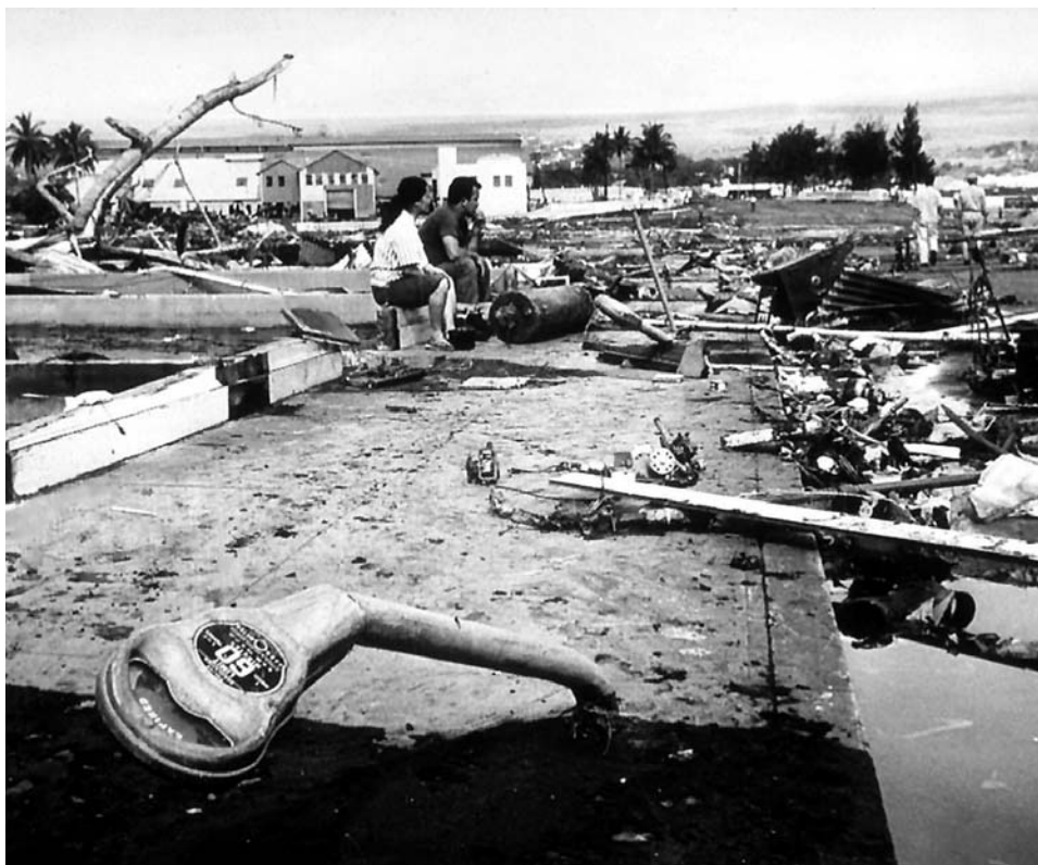
Figure 5.11. Aftermath of the May 22, 1960 Chilean tsunami in the Waiakea area of Hilo, Hawaii, 10,000 km from the source area. The force of the debris-filled waves bent parking meters. Photograph credit: U.S. Navy. Source: National Geophysical Data Center, http://www.ngdc.noaa.gov/seg/cdroms/Volcanoes/tif_24/648001/64800113.tif
