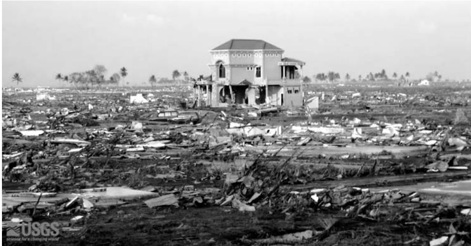
Figure 5.24. Total destruction of the urban landscape at Banda Aceh. Only houses and mosques made out of concrete were left standing. Source: Guy Gelfenbaum, U.S. Geological Survey. http://walrus.wr.usgs.gov/tsunami/sumatra05/Banda_Aceh/0730.html
