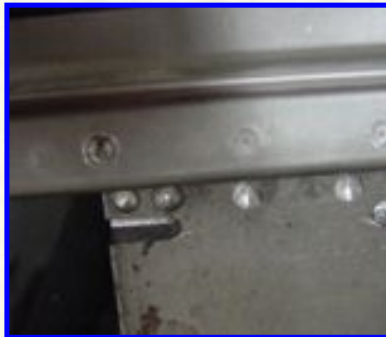
Rail support rivit installed
