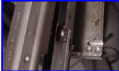
Rail support rivet, inside view
