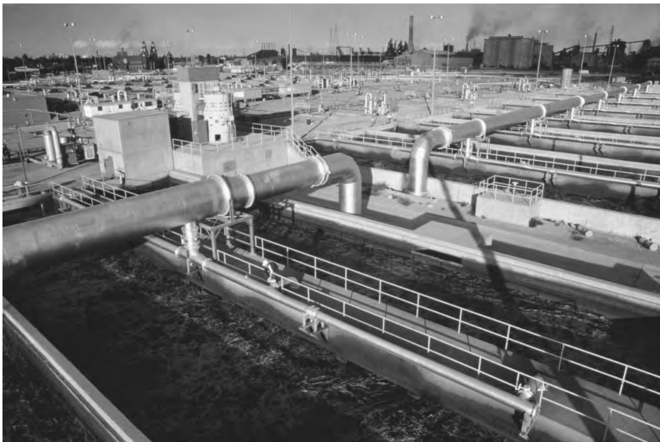
A wastewater treatment plant in Detroit, Michigan.
