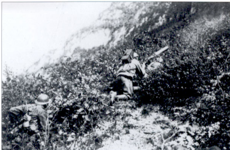
'Green Flames' in training exercises with a Fiat 14 machine gun, summer 1918. This particular firing style permitted the rapid movement of the weapon from one fire position to another, although it was a little awkward for the gunner who had to carry it. The troops might be from XXIX Reparto, which was based in Val Lagarina at that time. (MGR 21/456)
