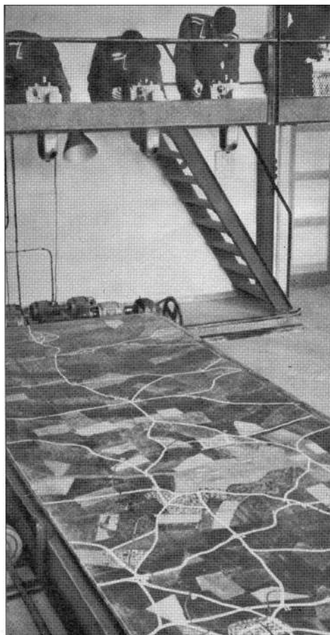
Trainee Beobachtere (observers) hold course over a motorized travelling landscape. Each must select and 'strike' various targets by pulling a wooden lever to his left, firing the bombsight camera shutter, and capturing an image with superimposed cross-hairs to verify his accuracy. Gearing enables instructors to complicate this task by applying realistic lateral drift. A defused lamp suspended beneath the gantry simulates moonlight for night-bombing exercises.
