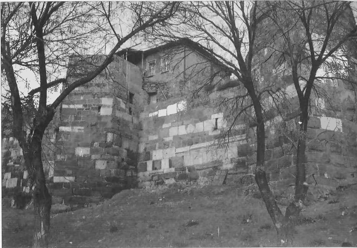
The walls of Ankyra were constructed around the year 900. Their pointed bastions are an unusual feature. Note the extensive use of recycled marble from earlier Roman buildings. (Author's Collection)
