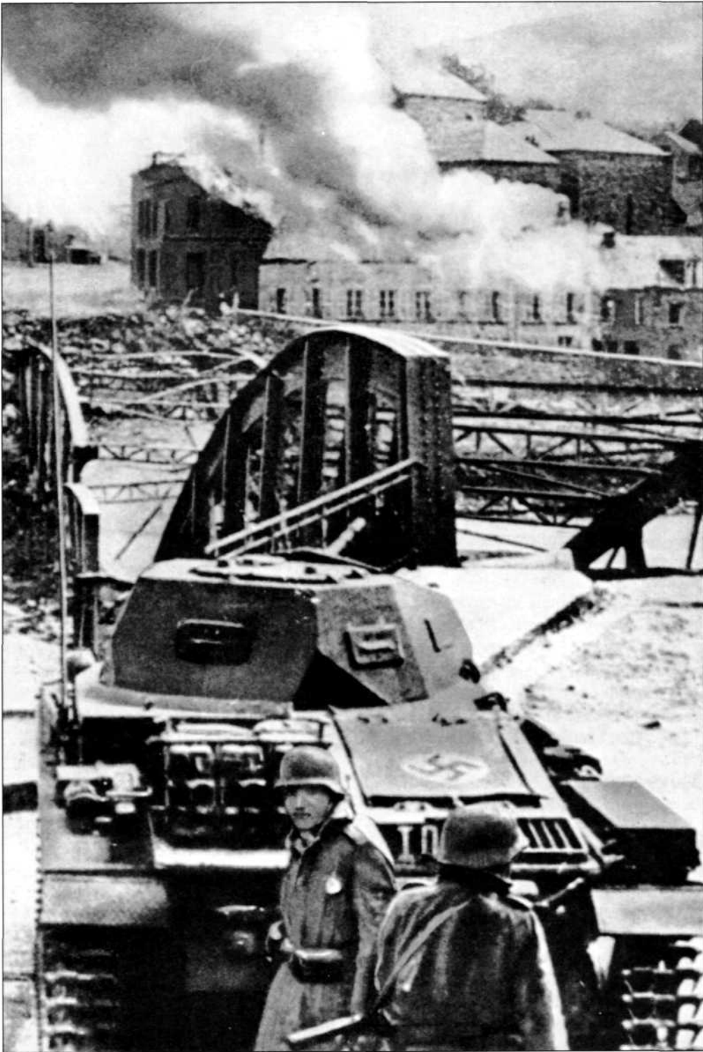
Blown bridge over the River Meuse. (Ann Ronan Picture Library)
