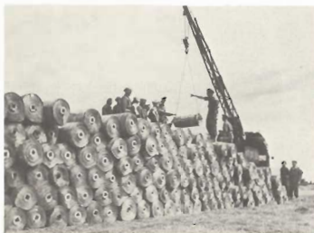
15. Landing strips in advanced areas were often laid using PBS—Prefabricated Bitumised Strips—over which went sections of perforated metal. A Coles Crane helps to stack PBS in a storage depot in France. (IWM)
