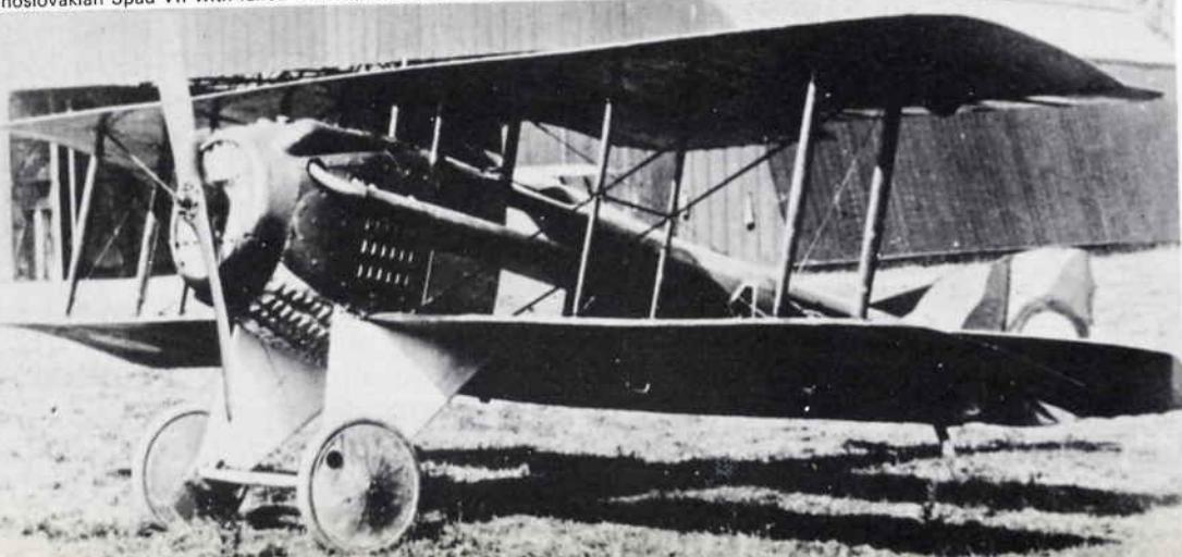
Below: Czechoslovakian Spad VII with faired undercarriage legs. (Photo: Zdeněk Titz).
