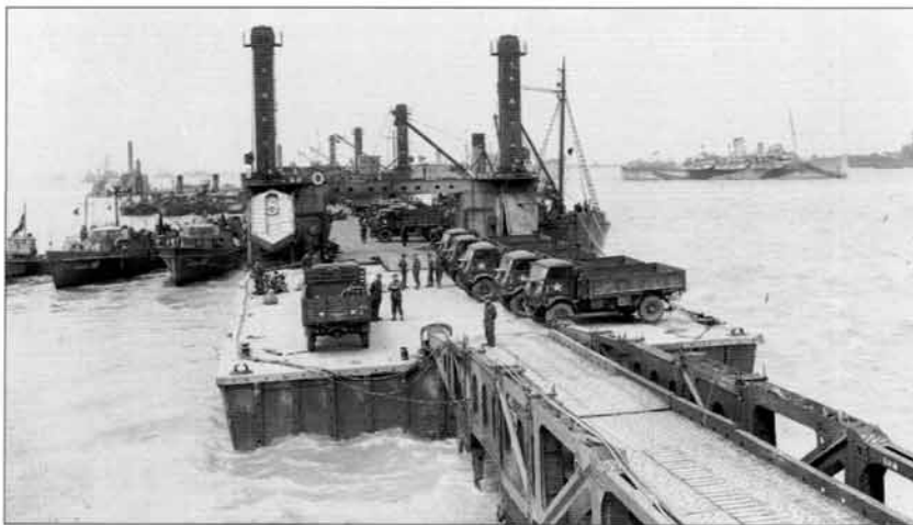
The pierhead of the British Mulberry artificial harbour at Arromanches. The harbour was damaged in the storm that began on 19 June, but was soon back in service and remained in use for the rest of the war. (IWM A24371)
