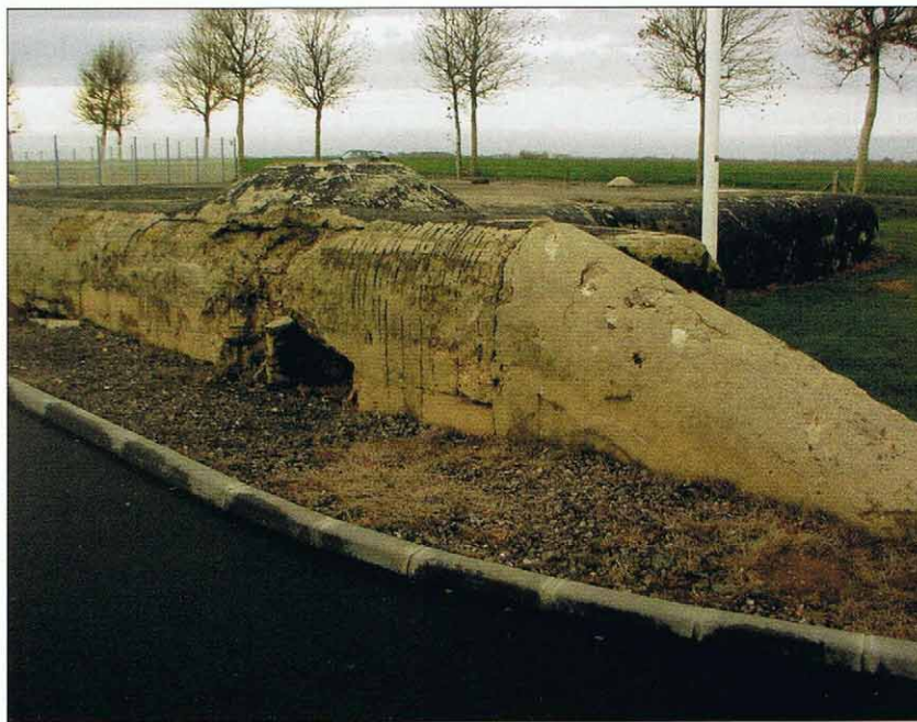
German command bunker near the present-day passenger terminal at Carpiquet airfield. Many of the concrete fortifications around the airfield had been constructed before the invasion and were strengthened after the landings to help defend Caen. The presence of these impregnable positions garrisoned by 12th-SS Panzer Division made Carpiquet and its airfield a formidable obstacle for the Canadians. (Ken Ford)
