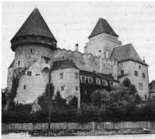
The Austrian castle of Heidenreichstein lay near the border with Bohemia. Lacking steep slopes, this important fortress made use of a moat, hence the name of wasserburg for castles built on such sites. Though begun in the 12th century the castle underwent many alterations; it was besieged by the Hussites, as well as by rebel peasantry in the 15th century. Notice the wooden hoarding on the round tower, which allows defenders to overlook the base of the wall; and the 13th-century watchtower or bergfried common in Germanic castles. (By courtesy of the Austrian National Tourist Office)
