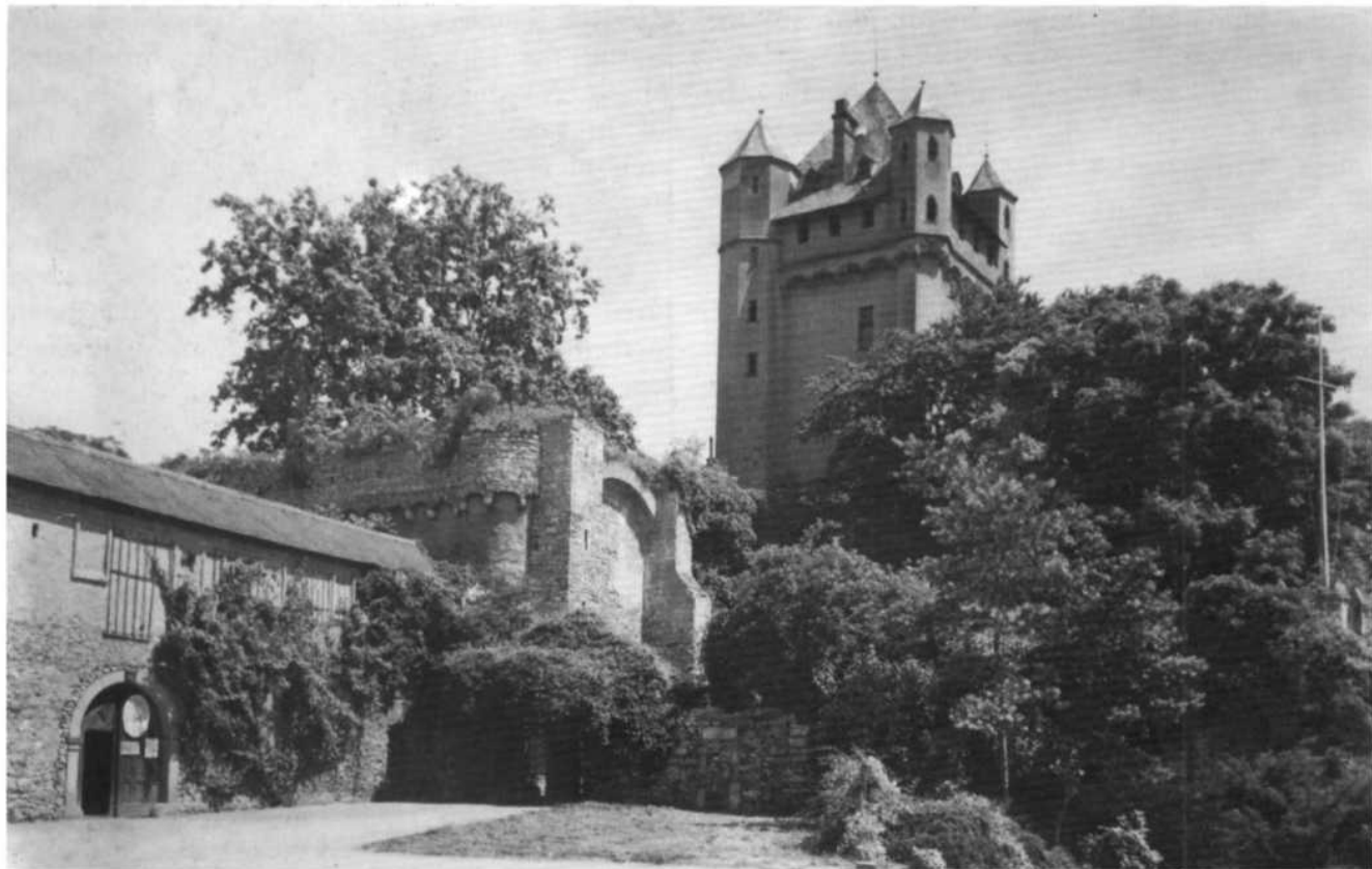
The castle of Eltville on the Rhine, built by Archbishop Baldwin of Trier in about 1330. During the 14th century some castles were built which followed more closely the trends established in Western Europe. These included regular ground plans, flanking towers, and, as seen here, the erection of tower houses. (Embassy of the Federal Republic of Germany)
