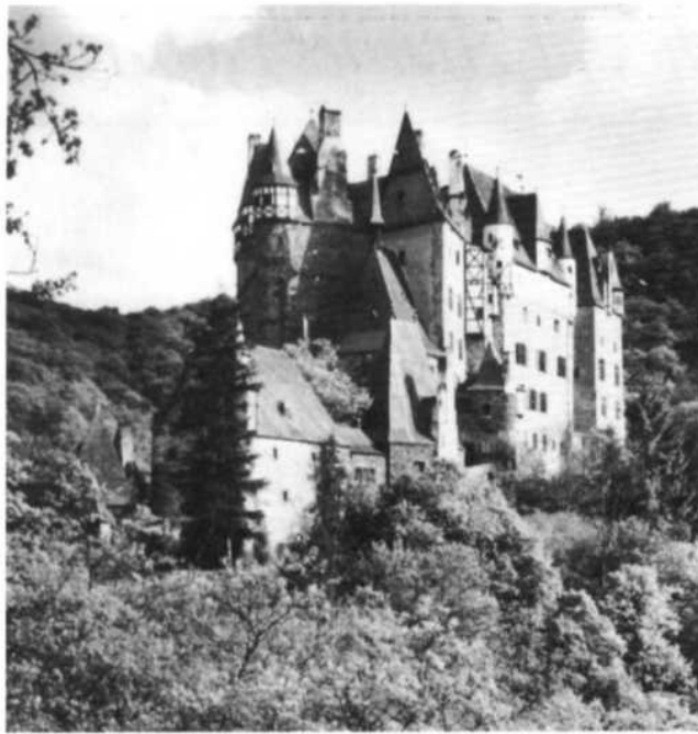
Eltz Castle on the Mosel. Many strongholds of the 14th and 15th centuries were basically earlier structures modified to meet the growing demands for comfort. The siting of numerous castles on near-impregnable crags or steep slopes resulted in irregular ground plans, while ranges of domestic buildings were amalgamated into the outer walls. (Embassy of the Federal Republic of Germany)
