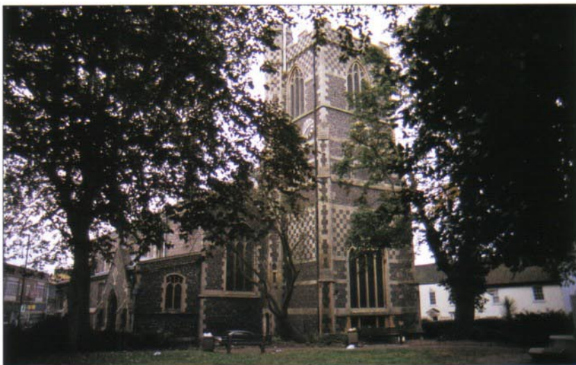
The church of St Mary the Virgin, Barnet, on the north side of the junction of the High Street with Wood Street. Yorkist refugees and Oxford's men must have swept past here during the rout of Hastings' division.
