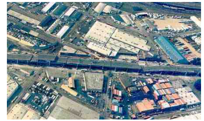
i / The collapsed section of the Nimitz Freeway
