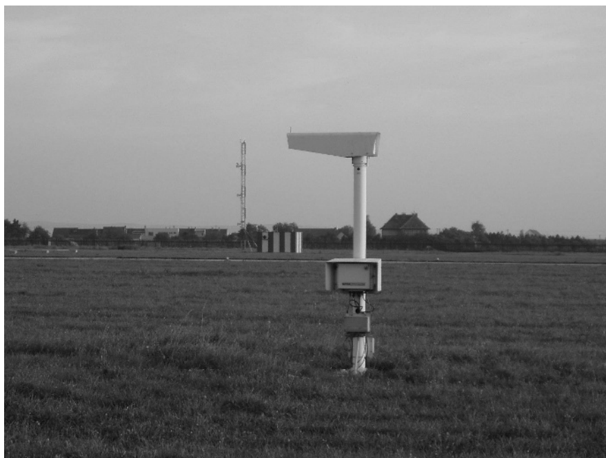
Figure 3-4 Part of RVR equipment in touchdown zone (ILS GP antenna behind) (Photo: A. Kazda)
