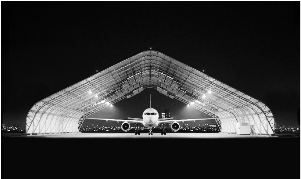
Figure 18-13 InfraTek de-icing facility of Radiant Aviation Services – RAS (Photo: Courtesy Oslo Airport)
