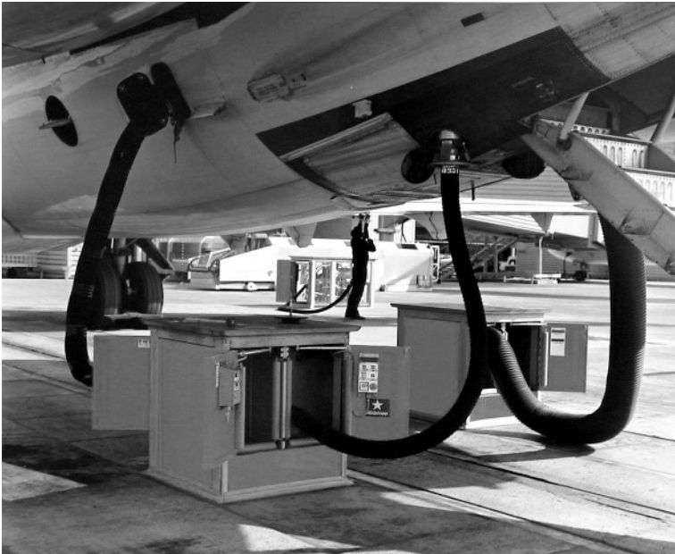
Figure 9-3 Fixed ground handling systems ‘vehicle free apron’ - FMT Pop-Up Ground Support System (Photo: Courtesy FMT - Fabriksmontering i Trelleborg AB)
