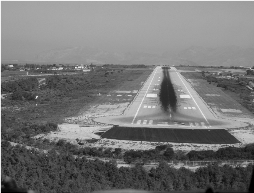
Figure 4-15 Turn pad at the runway end
