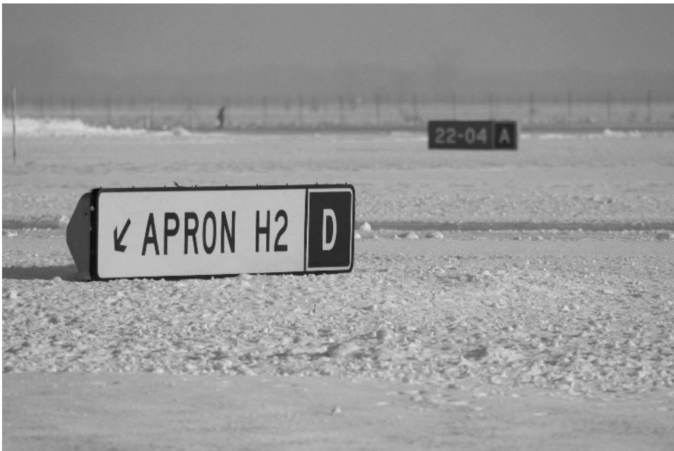
Figure 15-5 Information sign (left) and mandatory instruction sign (right) (Photo: Courtesy of Bratislava M.R. Štefánik Airport)
