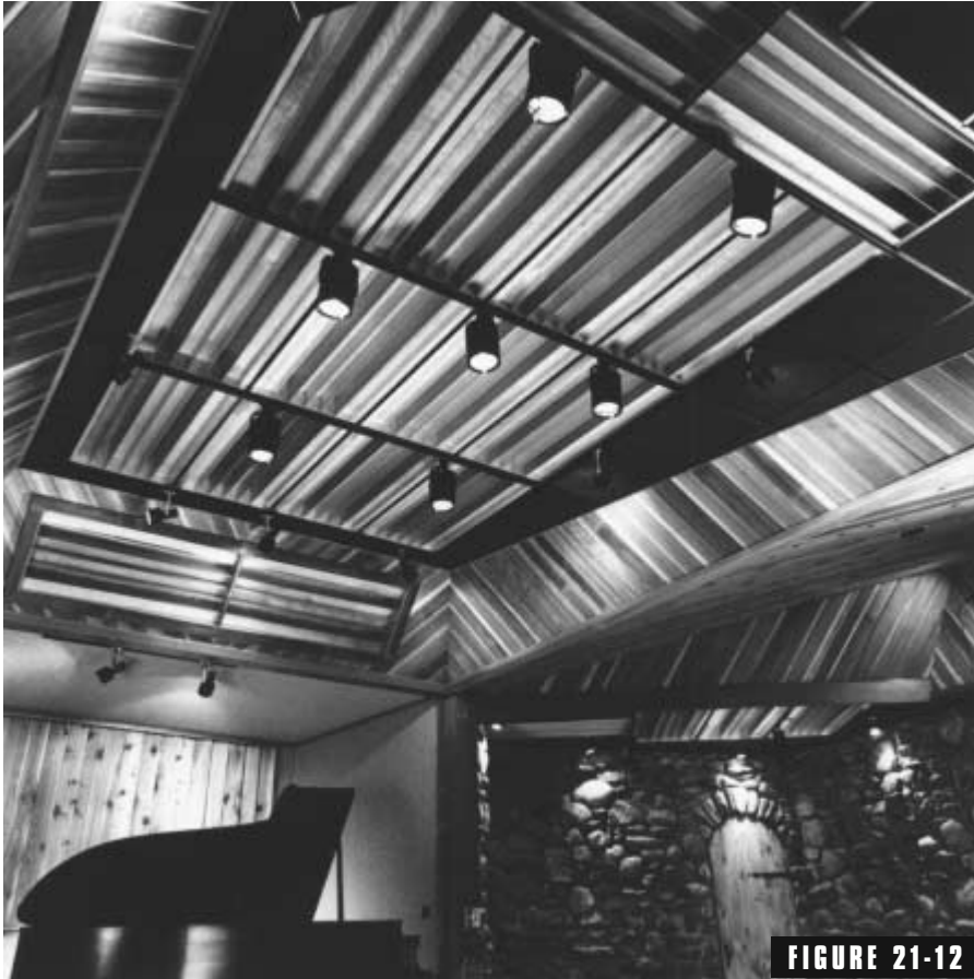
Blue Jay Recording Studio of Carlisle, MA, showing extensive use of RPG diffusers on the ceiling and elsewhere. Designed by Russell L. Berger, then of the Pelton-Joiner-Rose Group of Dallas, TX. Peter D'Antonio, RPG Diffusor Systems, Inc.
