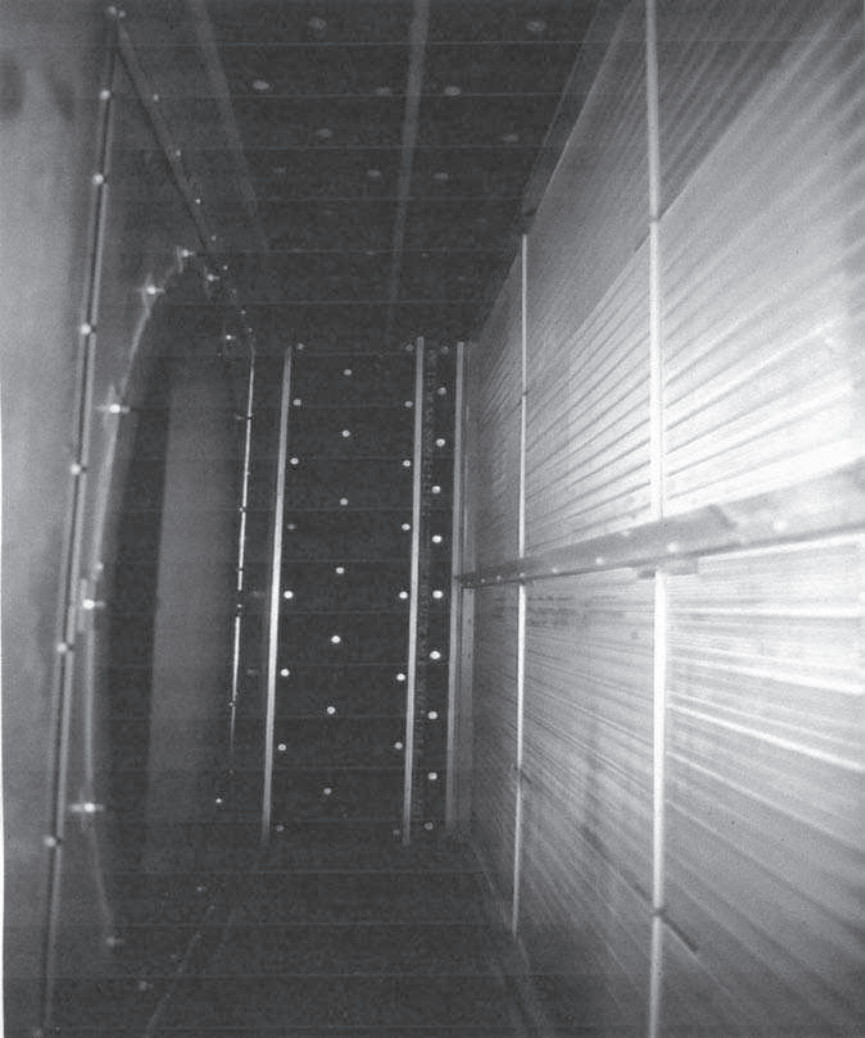
Figure 1-4. Hot Water Heating Coil
