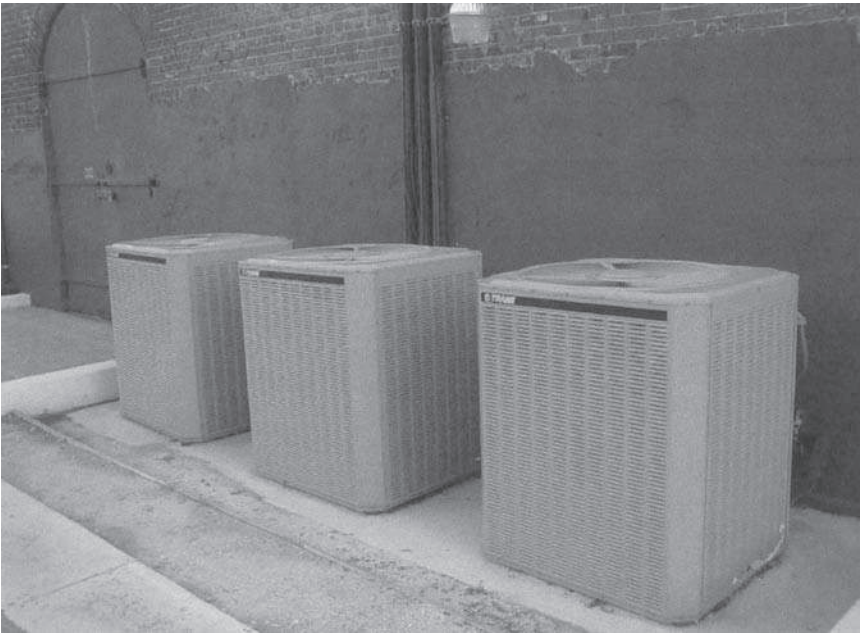
Figure 15-1. HVAC heat exchanger. Air-cooled condenser (refrigerant to air).
