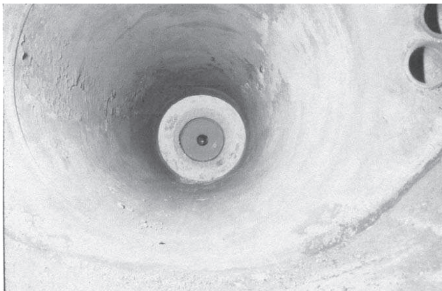
Figure 16-1. Inspecting firing chamber.
