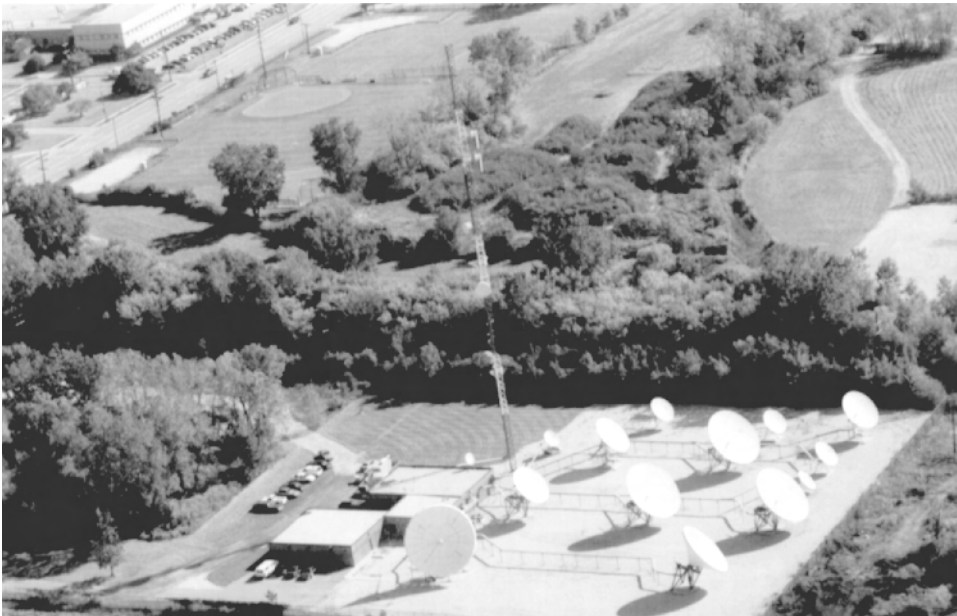
FIGURE 58.2 Teleport Chicago Earth station.
