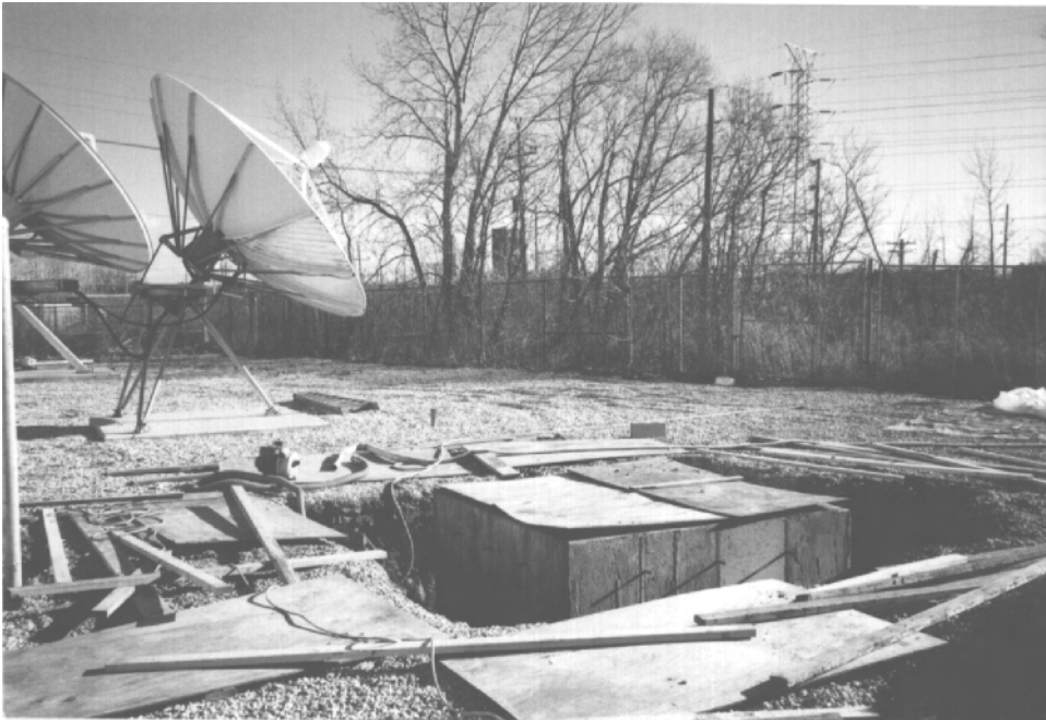
FIGURE 58.6 Antenna pad construction.
