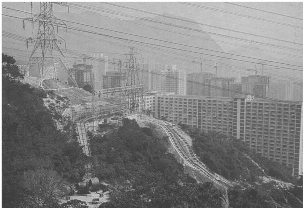
**Fig. 36.3** A bond pull route for 400 kV PPL cable which has a very steep gradient in addition to onerous bends at termination positions
