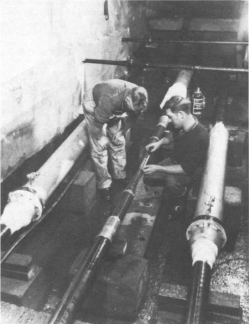
**Fig. 35.17** Joint bay for 275 kV fluid-filled cables
