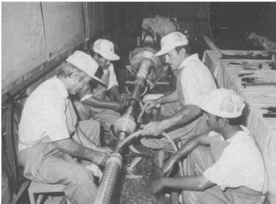
**Fig. 35.18** Joint bay with 275 kV stop joint for fluid-filled cable
