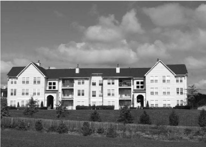
Figure 19-3: By choosing a piece of level ground some distance away to photograph this apartment complex, I was able to hold my camera level and avoid keystoneing.
