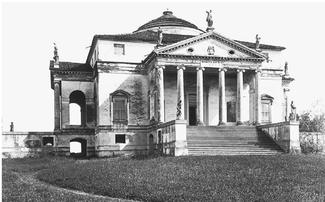
The Villa Rotonda, built by Andrea Palladio in Vicenza, Italy (1567-70). (Bettmann/Corbis. Reproduced with permission.)
