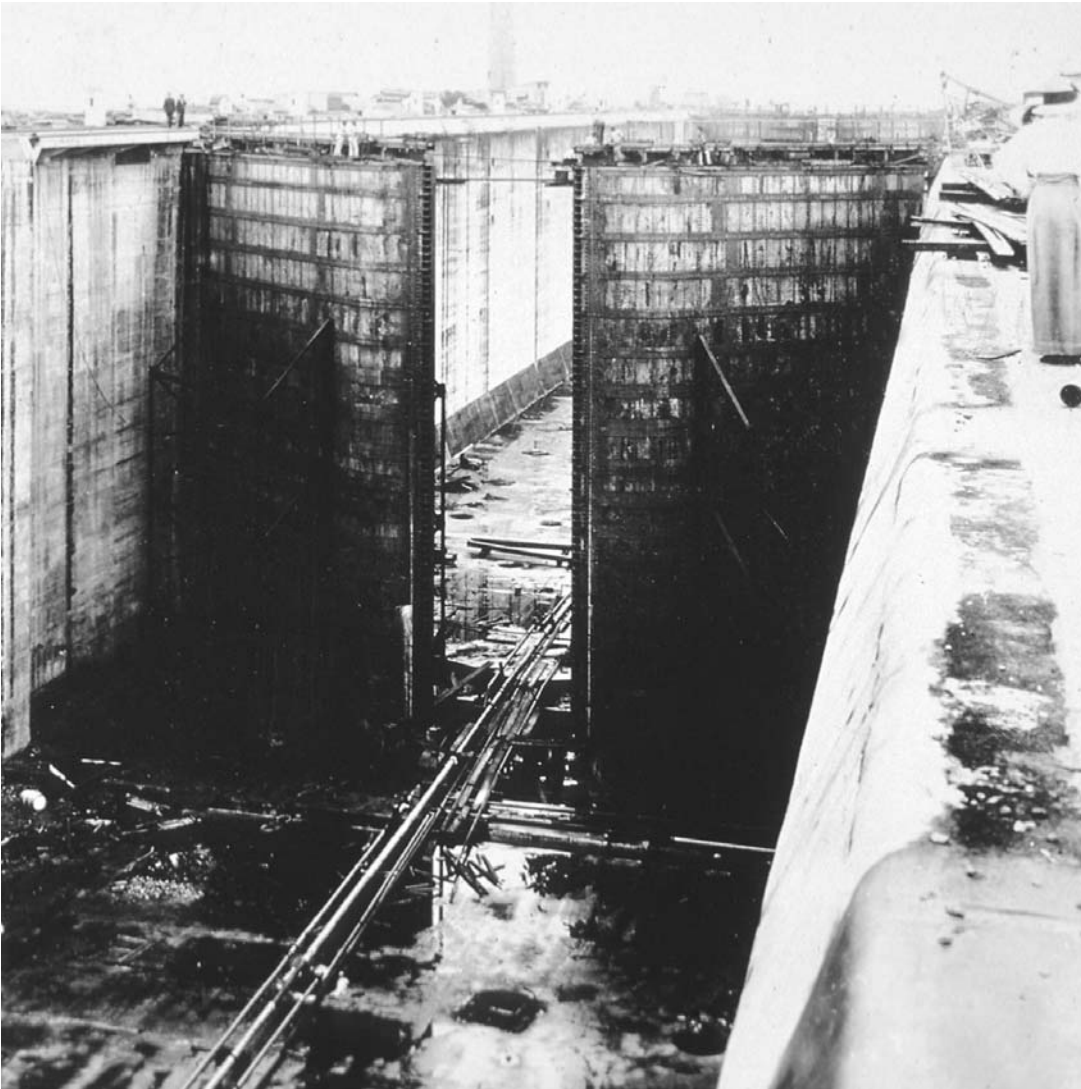
Panama Canal lock gates under construction (1913). ( Archive Photos. Reproduced with permission. )
