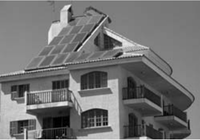
Figure 8.1. Solar electric panels. Courtesy of Painet.
