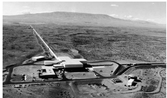
Figure 22.7. The LIGO detector at Hanford, in the US state of Washington. Each arm stretches 4 km, with mid-stations at 2 km. The arms house the world's largest vacuum system, inside of which intense laser beams monitor the separations between mirrors that are suspended in such a way that they are free to move along the direction of the arm in response to a gravitational wave. The system is able to sense motions as small as 4 \times 10^{-18} m if they occur in 10 ms. Image courtesy of LIGO.
