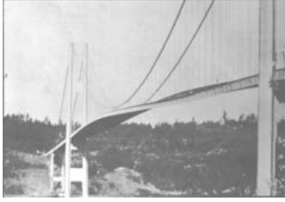
Figure 8.7. The classic example of the importance of normal modes in engineering is the Tacoma Narrows bridge disaster. The bridge was built across a waterway in the American state of Washington. Wind blowing across the bridge excited a normal mode whose pattern was a torsional oscillation of the roadway. The bridge became a tourist attraction on windy days, until a particularly strong wind drove the oscillations to a larger size than the structure could cope with. The roadway broke up on 7 December 1940. Reproduced with permission of the Smithsonian Institution.
