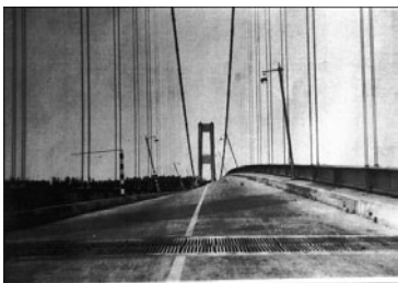
Figure 3.7 The Tacoma Narrows Bridge shortly before its collapse in 1940. The sidewalk to the right is over 28 ft above the one to the left.
