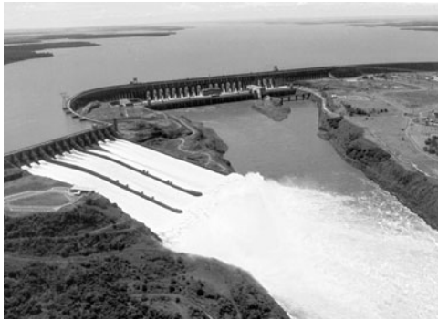
Figure 15.3 Spillway of the Itaipu Dam in Brazil.
