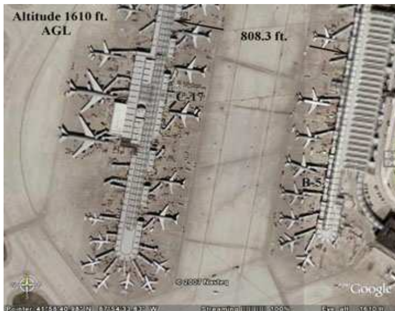
Figure 1. Aerial Photograph of United Concourses B and C from Altitude of 1,610 Feet.
