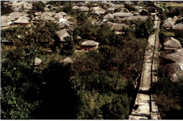
The outer wall of the Nagan Folk Village near Suncheon in Korea. Nagan is the best preserved of the walled towns defended against wako attacks. Its original earth wall was built in 1397, and replaced by a stone wall in 1424.
