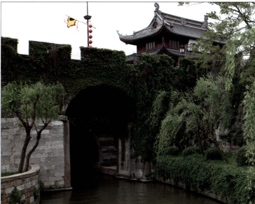
The Pan Men in Suzhou is a double water gate combined with a double land gate built against the Japanese pirates. Here we see the outer entrance to the water gate, which is defended by two stone portcullises that could be dropped across the canal.
