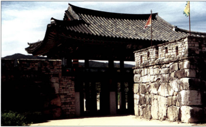
A defended gateway in the wall of Nagan Folk Village. Characteristic of Korean defensive architecture, the gateway is defended by a solid stone wall that extends outwards to oblige an attacker to make a 90 degree turn.
