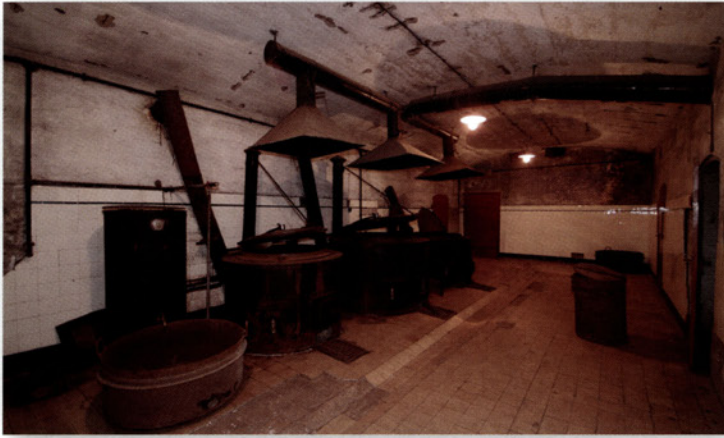
The kitchen of Infanterie-Werk Avigy, Feste Wagner, with three steam pressure cookers and a hot water heater on the left for tea and coffee. (Dan McKenzie)
