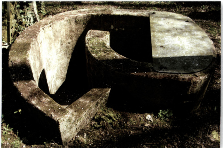
A concrete ‘snail’ sentry post. Many of these were built of sheet metal and scattered throughout the perimeter defences of the Festen . The roof provided protection from small-arms fire. Note the visor in the right foreground. (Author’s collection)
