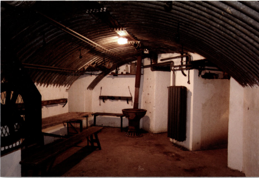
A forward troop assembly shelter near one of the exits to the infantry parapets. The undulating sheet metal ceiling prevented concrete dust from falling on the troops and equipment. (Dan McKenzie)
