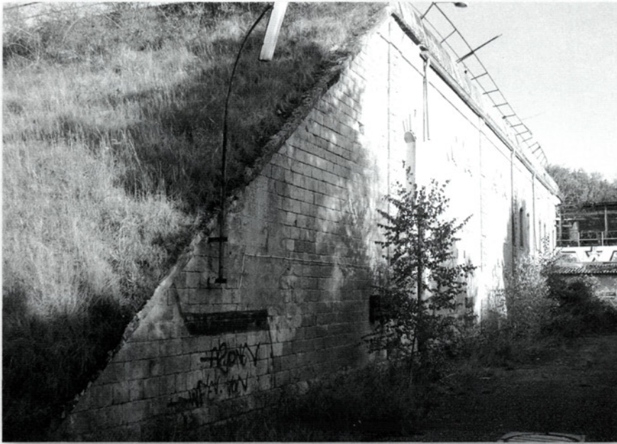
Barracks 4 of the Feste Kaiserin (Groupe Fortifié Jeanne d'Arc). In the background is the defensive caponier with a modern addition on top. This building was used by NATO forces from the 1950s to the 1960s as an air traffic control facility for north-eastern France. (Author's collection)
