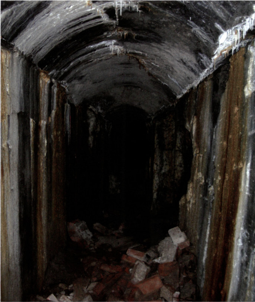
The tunnel in which several days of fighting took place between US and German troops in the battle for Fort Driant in October 1944. The tunnel connected Barracks R in the south-east corner of the fort with the 15cm armoured battery. (Author's collection)
