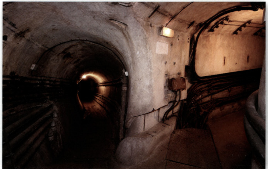
An oval-shaped tunnel at Feste Guentrange. (Mark Bennett)
