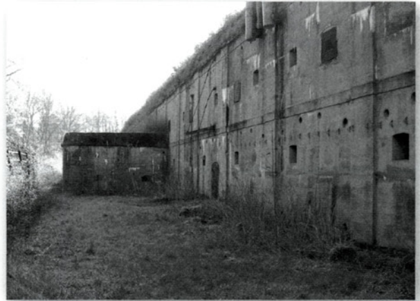
The barracks of Infanterie-Werk Verny, Feste Wagner. The gorge ditch was defended by 5.3cm guns in the central caponier jutting out from the face of the building. (Author's collection)
