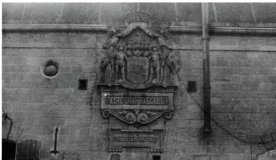
The barracks of Fort St Blaise of Feste Graf-Haeseler. The family crest of that family is above the entrance. The façade is of yellow stone, the original material used in construction. To the right is a chimney for the heating stoves. This was heavily damaged in 1944. (National Archives and Record Administration)
