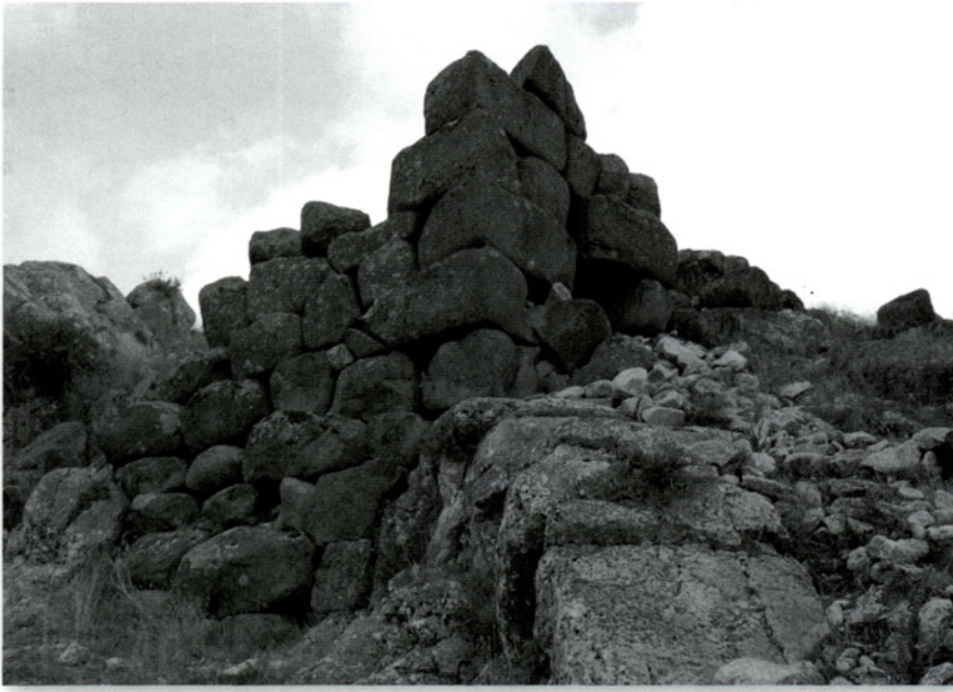
Gavurkalesi. The remains of a Hittite fortification wall made of huge andesite blocks without mortar. Most of the stone blocks are 120–150cm long and about 50cm high.
