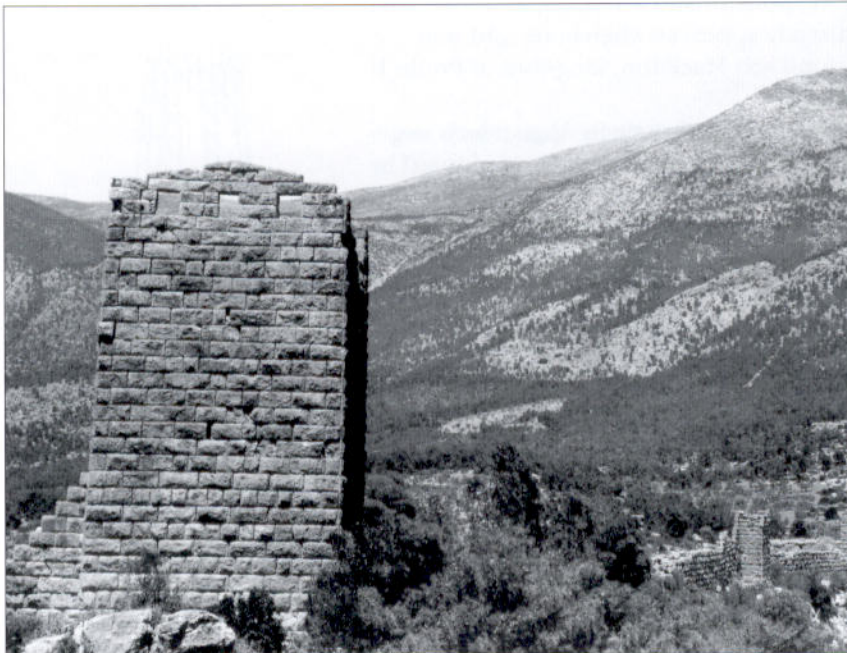
A tower from the fortifications at Aegosthena, thought to have been built by the Athenians around 343 BC. The top floor is often said to have accommodated catapults, because it has three windows (approx. 0.8 x 1.1m) per side. (A. W. Lawrence, courtesy of the Conway Library, Courtauld Institute of Art)
