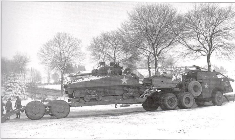
One of the more conspicuous pieces of equipment in the armored division was the M25 "Dragon-Wagon" tank transporter consisting of the M26 tractor and the M15 semi-trailer. There were nine of these in each division's ordnance maintenance battalion. The powered winch assembly behind the cab allowed them to retrieve damaged medium tanks as seen here as a knocked-out 4th Armored Division M4A3 tank is recovered near Bastogne on January 6, 1945, ten days after the division relieved the besieged town. (US Army)
