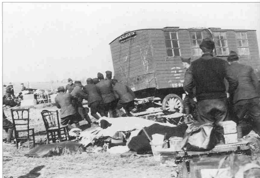
Telegraph trailer at First Army headquarters, Souilly, France, being moved out of danger from incoming fire during the Meuse-Argonne campaign, October 30, 1918. (US Signal Corps, 28413)
