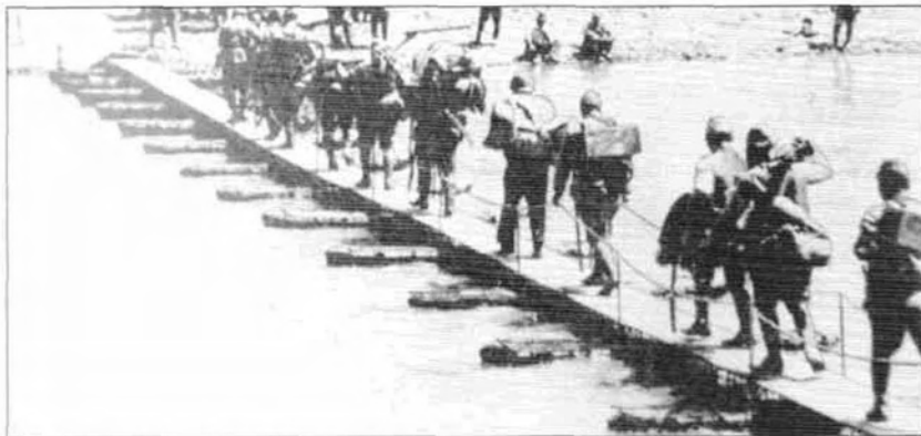
The Japanese forces were fairly well equipped with light bridging and bridge-repair matériel. They recognized the necessity of maintaining the speed of offensive operations through difficult terrain.
