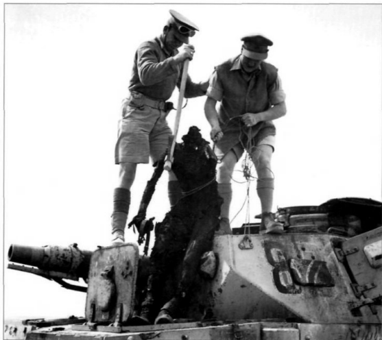
The burnt remains of the radio-operator of a German PzKpfw IV tank is hoisted out of his compartment, 30 March 1942. (4700-32 E 9986)
