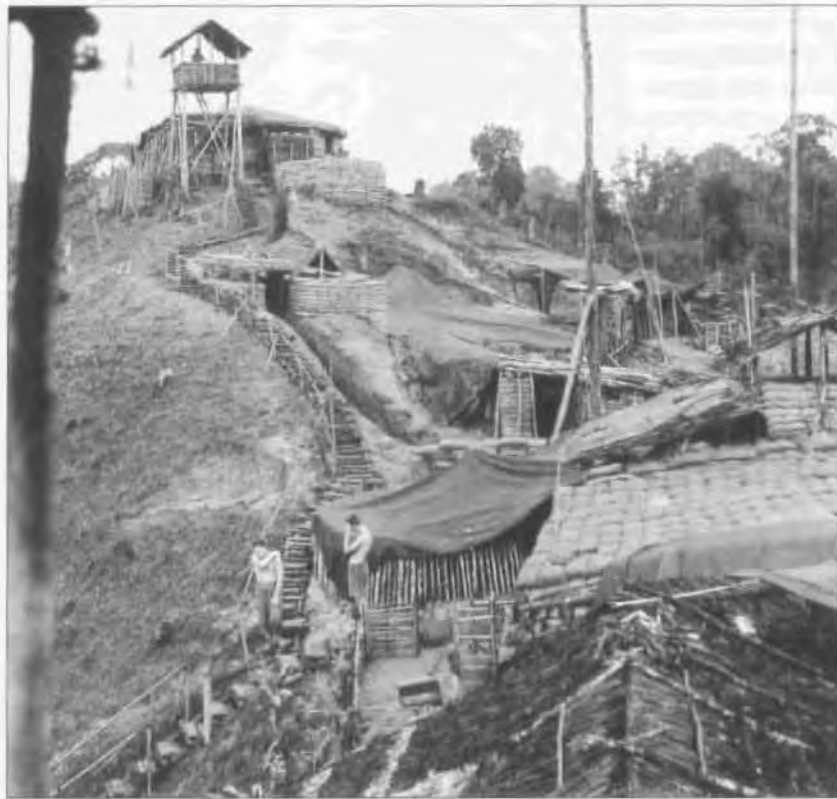
A typical border fort in Sarawak. It has an observation tower, bunkers made of logs and sandbags linked by communication trenches, and a stepped walkway up the hill – essential in the muddy conditions created by tropical rainfall – made of cannibalized ammunition boxes. Note the tall poles supporting radio aerials, and the vegetation cleared away to provide good fields of fire. (IWM FES 64/242/4)
