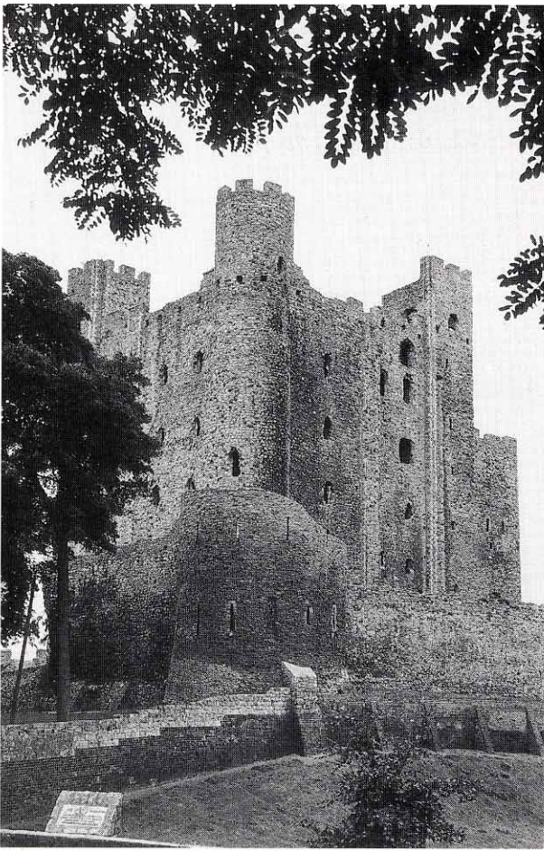
Rochester castle, Kent, a large keep and forebuilding built in Kentish rag by William of Corbeil in c. 1127. The single round corner turret bears witness to the siege of the barons by King John for almost two months in the autumn and winter of 1215, when royal miners breached the outer wall and drove a mine under the keep. Having filled the cavity with wooden props and pig fat, the whole was fired and the corner collapsed. Even then the defenders retreated behind the great cross wall, which divided the keep internally, and continued to resist. When rebuilt, the corner was given the present rounded face, which left no sharp corners for sappers.
