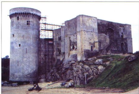
Falaise castle seen from the courtyard, showing the donjon's first-floor entrance, now masked by a modern forebuilding. Philip's tower is clearly visible.
