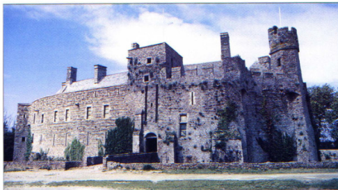
The small castle at Pirou is a simple enclosure with no donjon. The walls are probably of late-12th century date. A single polygonal turret survives, carried on large buttresses. Where these buttresses meet the wall, a triangular machicolation is formed. One can be seen on the far right of this picture.
