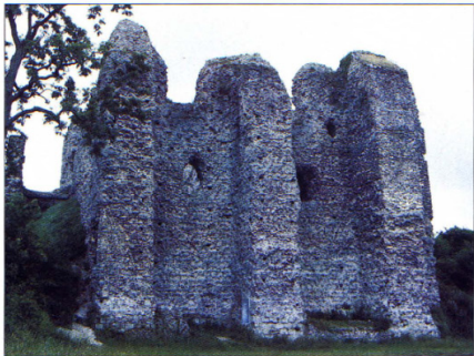
The donjon at Arques was provided with deep buttresses, shown here.
