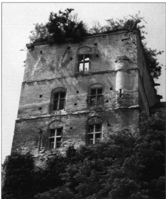
The square residential tower at the eastern corner of Tancarville castle was built in the 12th century, but the windows were altered and enlarged in 1360.
