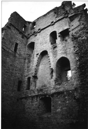
The interior of the donjon at Vire. The fireplace on the right has lost its stone hood.
