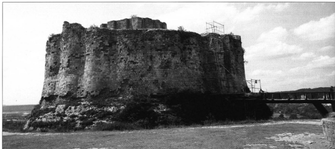
The inner corrugated wall at Château-Gaillard, seen from the middle bailey.
