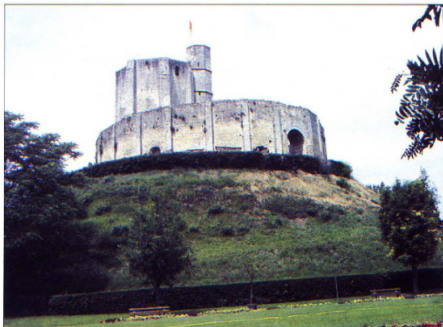
The motte at Gisors, showing the buttressed polygonal shell wall and the donjon.
