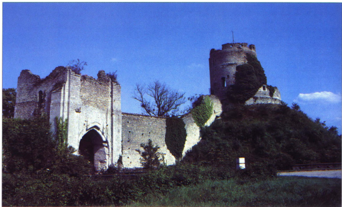
Château-sur-Epte is a motte and bailey castle in the Vexin, which was fortified in stone in the early-12th century. The gate-tower had drawbridge beam slots added in the 14th century. The cylindrical donjon on the motte rising behind the chemise was probably built by Henry II in 1184.
