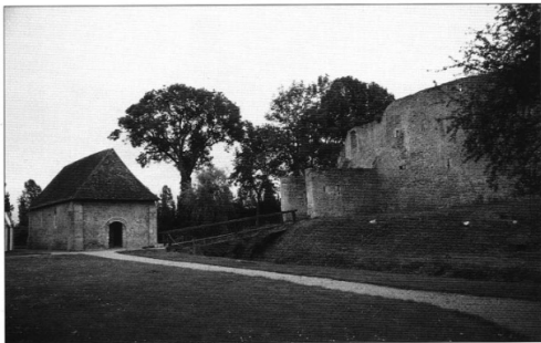
The 11th–12th-century chapel at the castle of Crèvecœur-en-Auge, with the bridge to the inner courtyard on the right.
