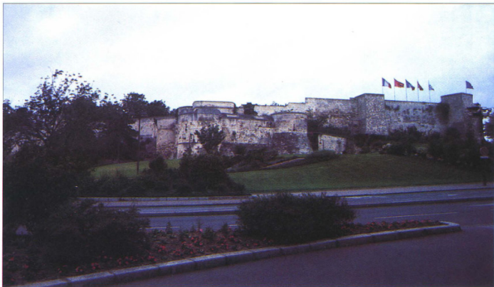
The walls of Caen have been altered over the centuries but still retain the essential line of Duke William's castle of 1047. Some of the rectangular towers may be of late-12th-century date.
