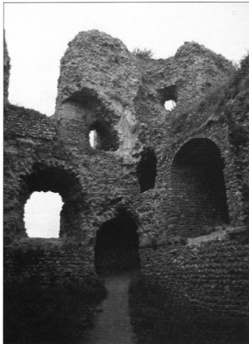
The interior of the donjon at Arques, showing the door leading to the passage to the curtain wall.
