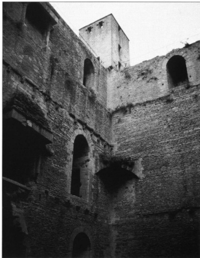
The interior of the donjon at Chambois. The timber floor beams were carried on stone corbels, visible along the walls.
