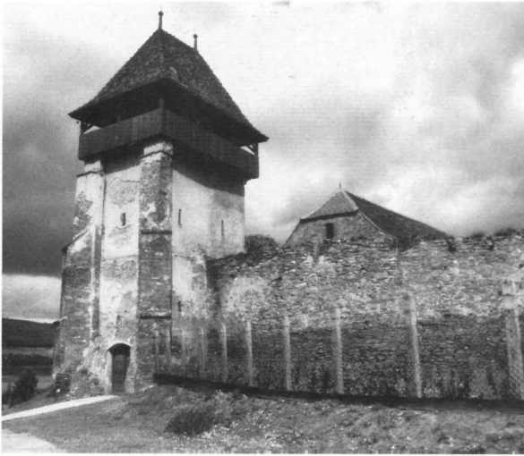
Gate-tower and surrounding wall of a church west of Medias. Many Transylvanian villages had such fortified churches serving as places of refuge in a war-torn region. Here the church lies within a curtain-wall with a tall tower above its only entrance.
