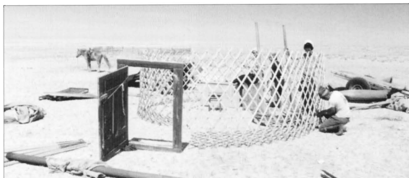
Erecting a ger. The framework of the walls was carried on pack animals and was opened up like a trellis. It was then pulled into a circle to create the wall of the ger. A number of straight poles were then fitted in around the upper rim of the side wall and joined at the apex by a circle that provided the smoke hole. (David Sneath)
