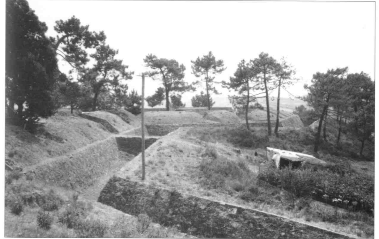
Fort San Vicente, Torres Vedras. A fine view of the ditch, glacis and the ramparts of the fort. Note the shape of the fort. It was constructed in such a way as to cover the approaches, and is a fine example of the way in which engineers turned away from the elaborate star-shaped forts of the previous century. The ditches and interior walls have been somewhat artificially preserved with concrete. It serves as a focal point for commemoration of the Lines of Torres Vedras.
