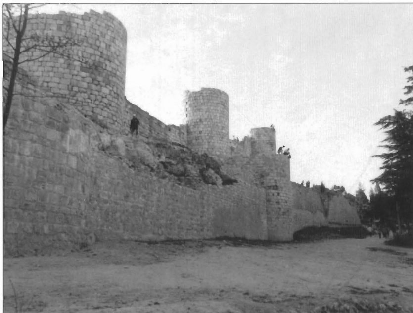
The strong walls of the eastern side of the castle of Burgos are pictured here. No attacks were made against this section of the walls.
