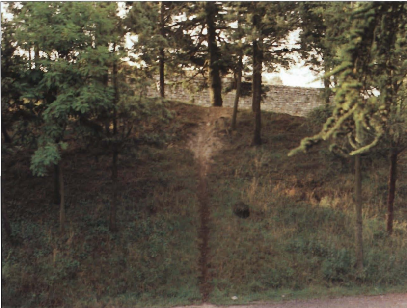
The massive bank of the third line of defences at Burgos, seen from the north. Behind the line the walls of the castle itself can just be seen.
