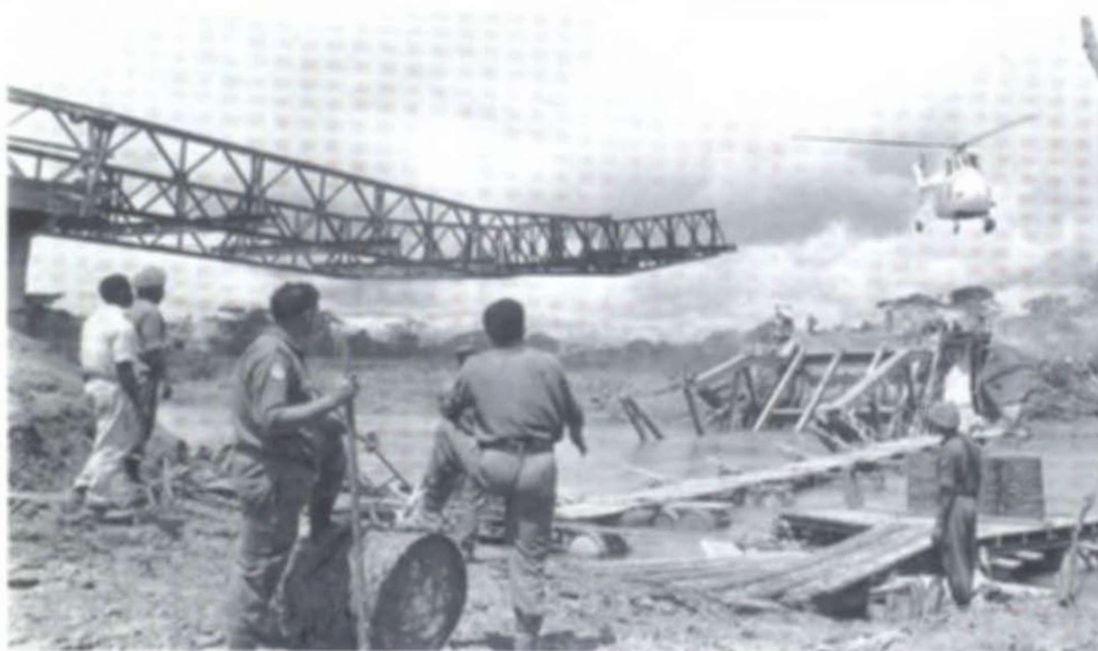
ONUC troops at a bridge over the Lufira River constructing a provisional bridge using empty oil drums to enable troops to continue operations; Katanga, January 1963. (United Nations)
