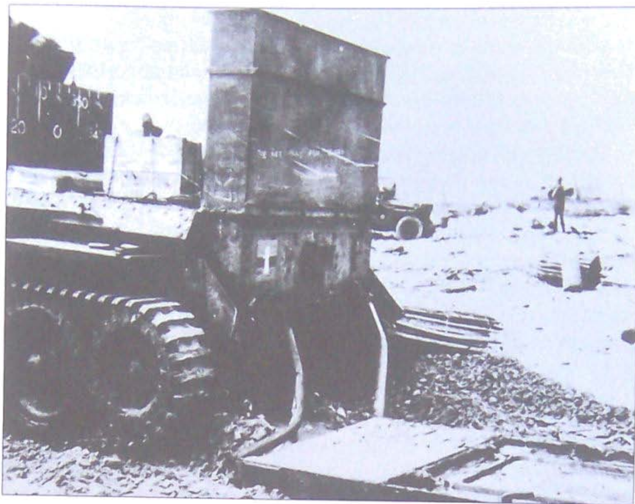
Abandoned on Gold Beach on D-Day, this Centaur of 1st Armoured Support Regiment, Royal Marines, has been selected to display the Deep Wading trunking and the Porpoise reserve ammunition sledge that it towed ashore behind it.
