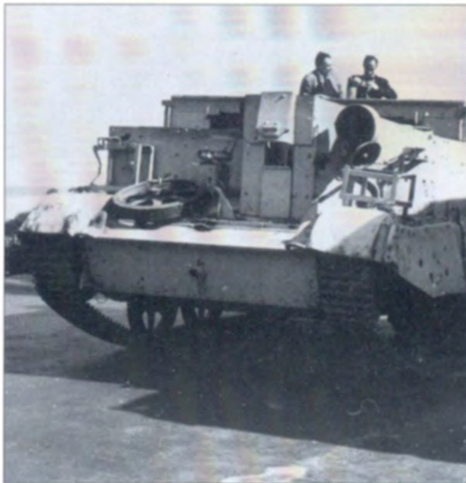
Abandoned by its current owners, a Universal Carrier of the Egyptian Army is examined by British troops during the 1956 Suez Crisis. Improvised sand shields, running full length, have been added behind the original valances.
