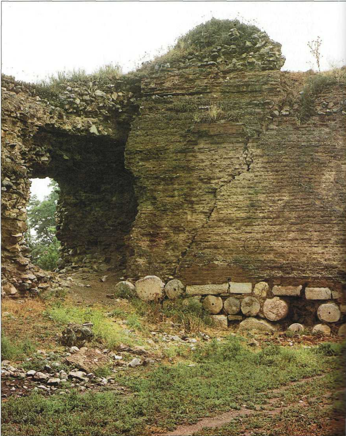
The walls of Nicaea, (modern Iznik, Turkey); the column bases and other reused material at the bases of the towers reflects their rapid construction. (Author's collection)
