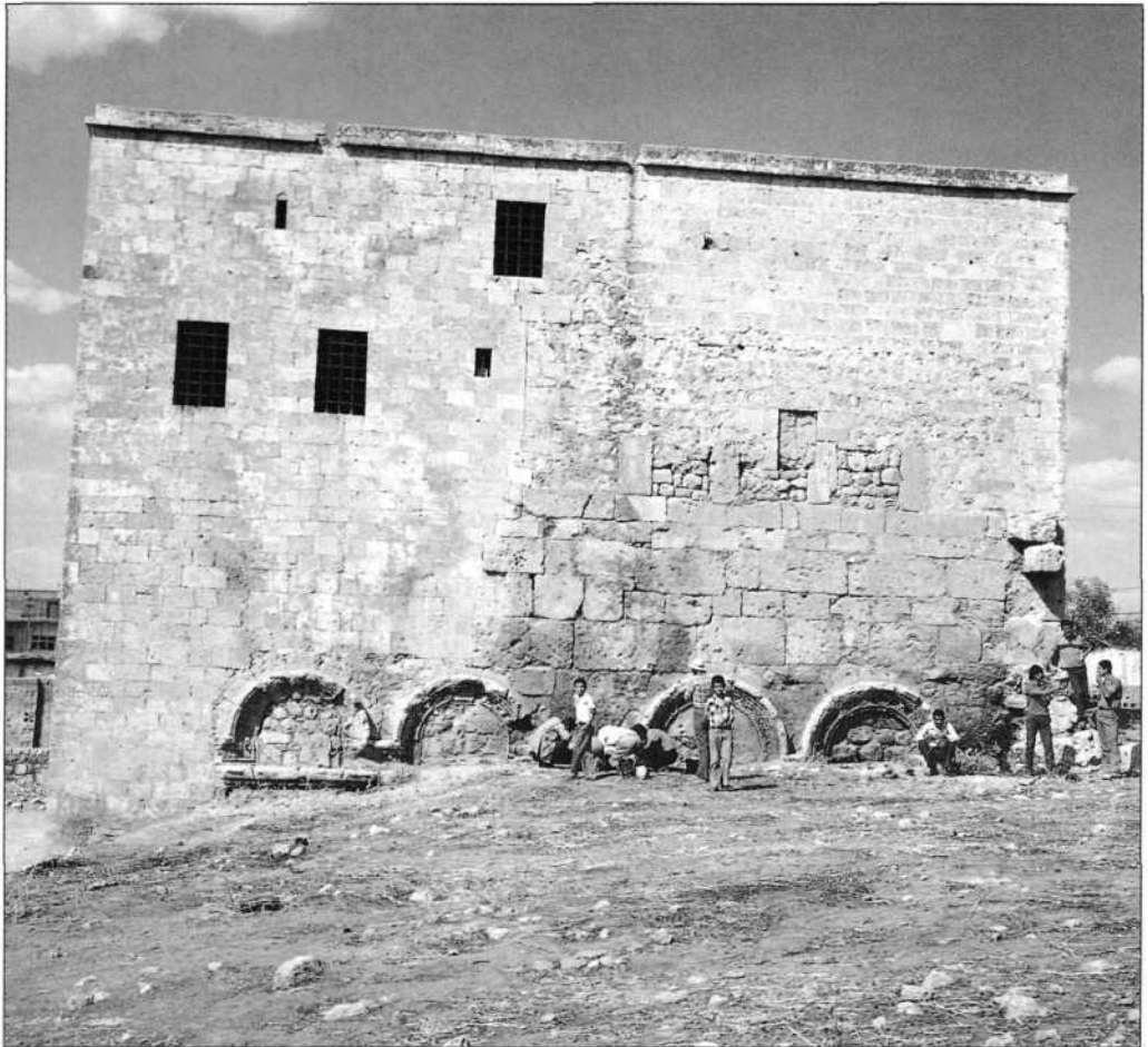
The Baptistery at Nisibis with the lintels of the original doors just visible. Only a year after the building's dedication Nisibis was transferred to Persian control by Jovian (AD 363). (Author's collection)
