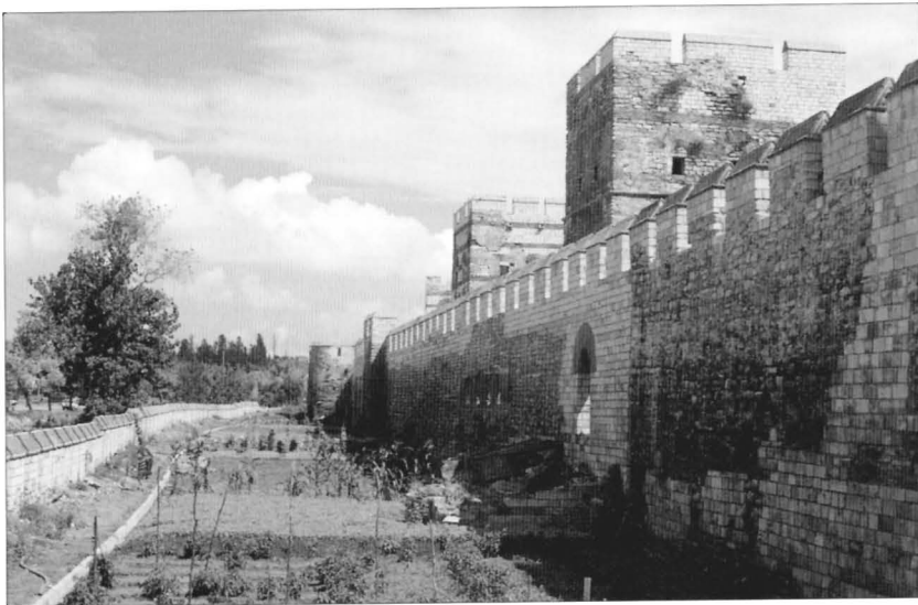
A restored section of the outer wall near the Belgrade Gate, showing the outer walkway, towers and a gateway.
