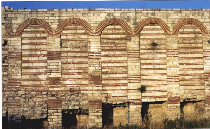
The Theodosian walls were constructed using stone and brick. In this detail of the sea wall on the Sea of Marmara both materials can be seen. Brick was used more sparingly than stone.
