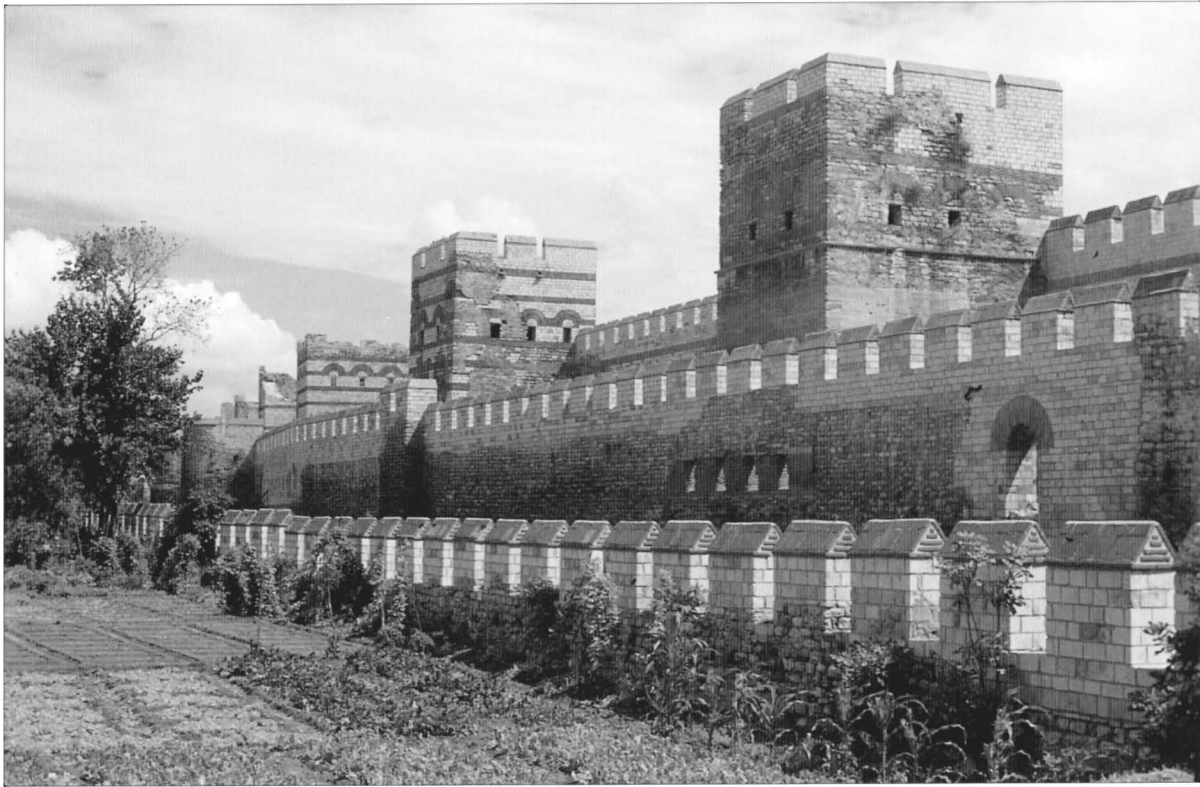
Possibly the finest restored section of the Theodosian walls lies here to the north of the Belgrade Gate. The complete system of inner wall, towers, peribolos , outer wall, outer walkway, small parapet and moat are shown here.
