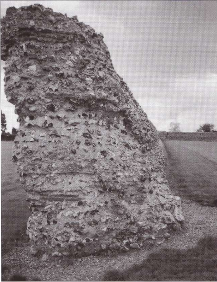
The inner faces of the thick, freestanding curtains of Burgh Castle- Gariannum are not vertical, being tapered as they rise. This view, looking south, shows the east wall running from the east gate. Note the lack of an earthen bank behind the wall. (Author's collection)
