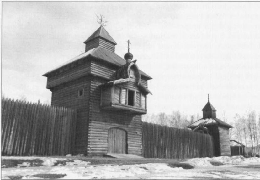
Gate tower of a mid 17th-century Russian wooden fortress, as reconstructed at the Taltsui Architectural & Ethnographical Museum. (Photo V.V.Tikhonov)
